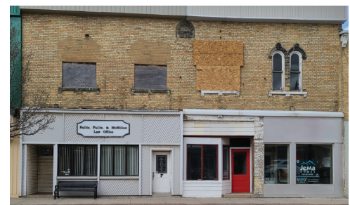
McEWING'S BLOCK, PALMERSTON Before CIP Grants (2020)
